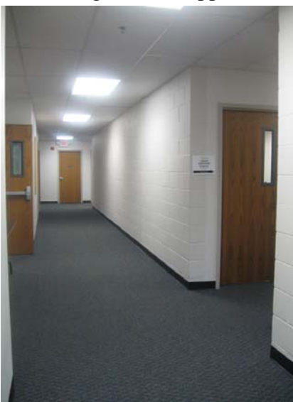
The blank walls of the 3rd floor
